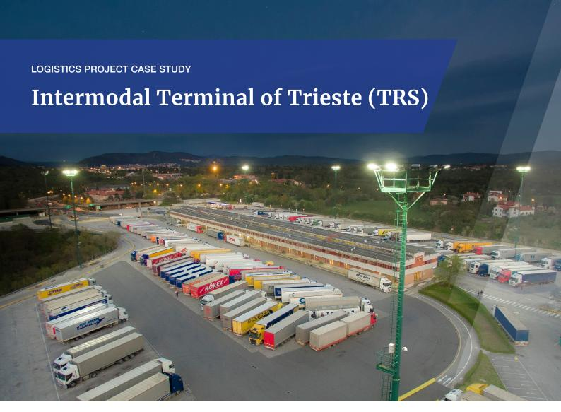
As with most intermodal terminals, TRS operates 24/7. So, lighting is critical. Traditional High Pressure Sodium lighting systems are costly to maintain and offer poor colour rendering for CCTV systems. Another reason for switching to LED lighting is to reduce neighbourhood light pollution. TRS asked us to upgrade their lighting to make sure it was delivering exactly what was needed for an intermodal terminal.
